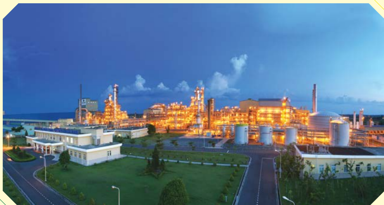
Overview of Ca Mau Fertilizer Plant in Ca Mau Gas – Power – Fertilizer Complex
