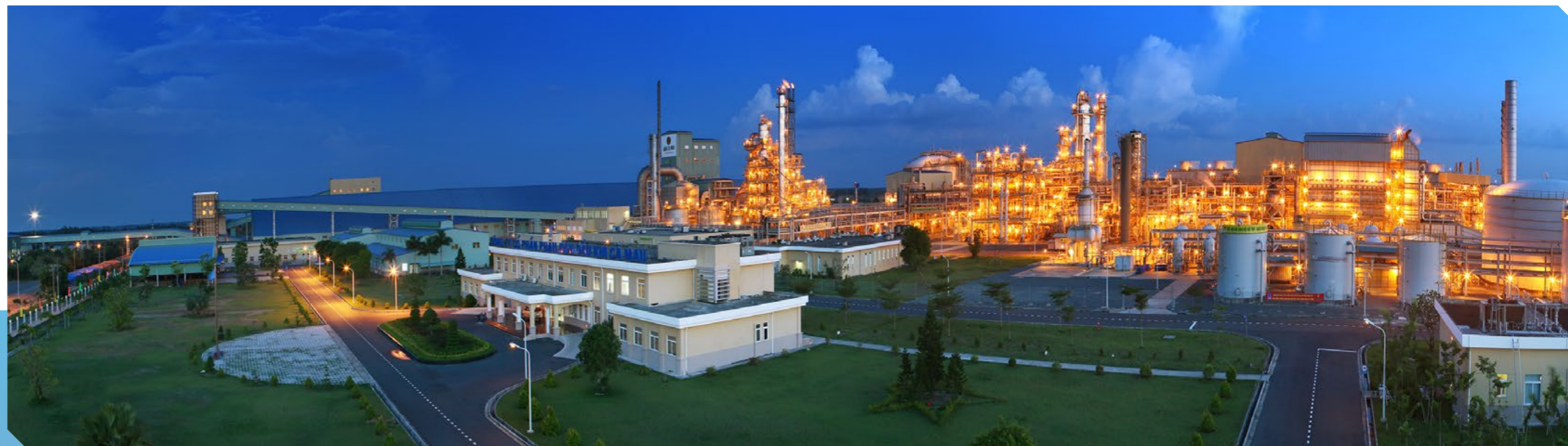
Overview of Ca Mau Fertilizer Plant
